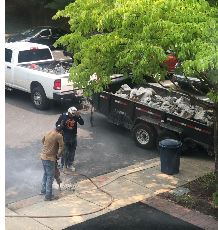
Concrete Replacement Project (Curbs, Gutters, Sidewalks)
