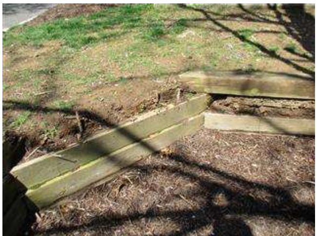
18 Tree Well/Planter (rotted wood, exposed rebar/steel bars) (March 2020)
