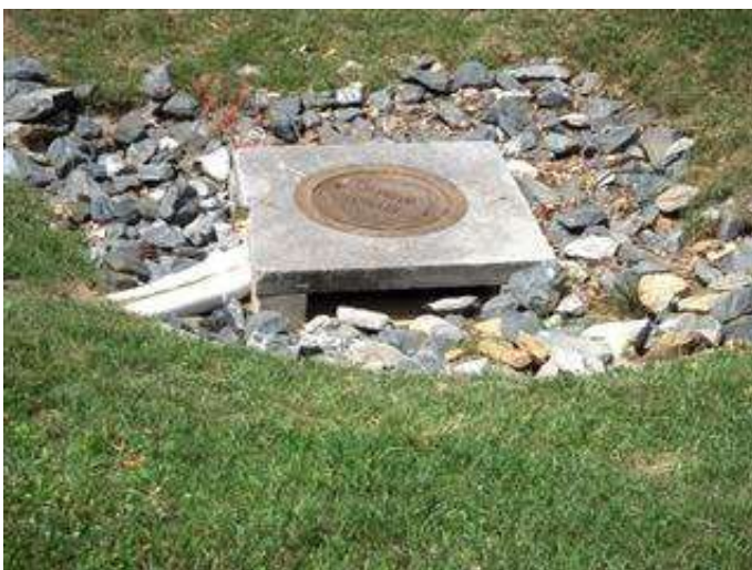
23 Stormwater Drain (near Tot Lot) (June 2024)
