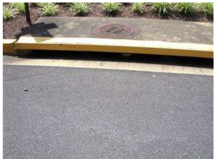
24 Stormwater Drain (at front entrance) (June 2024)
