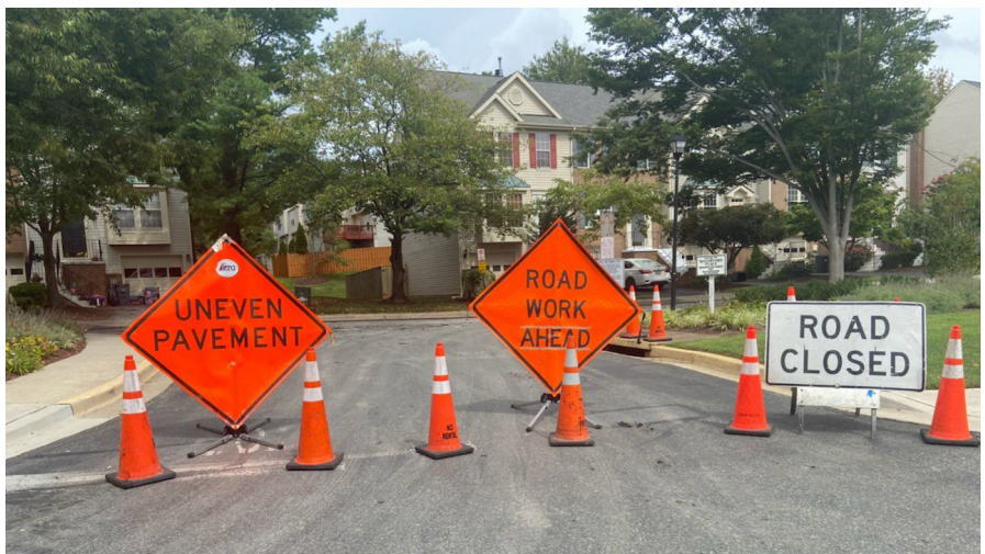
Waters Row Terrace Asphalt Resurfacing Project
